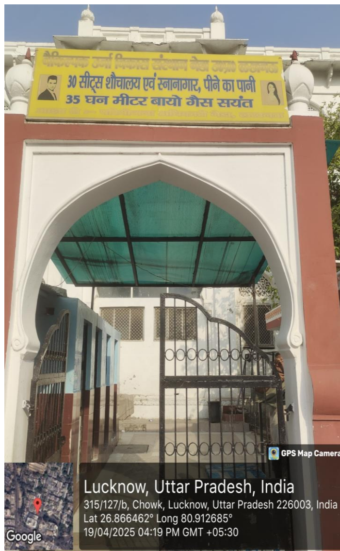
Sulabh Shauchlaya Complex located at KGMU
