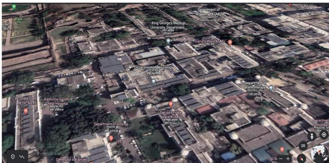
fig . Google Earth View of the Solar PV Panels Installed on various buildings within KGMU Campus
