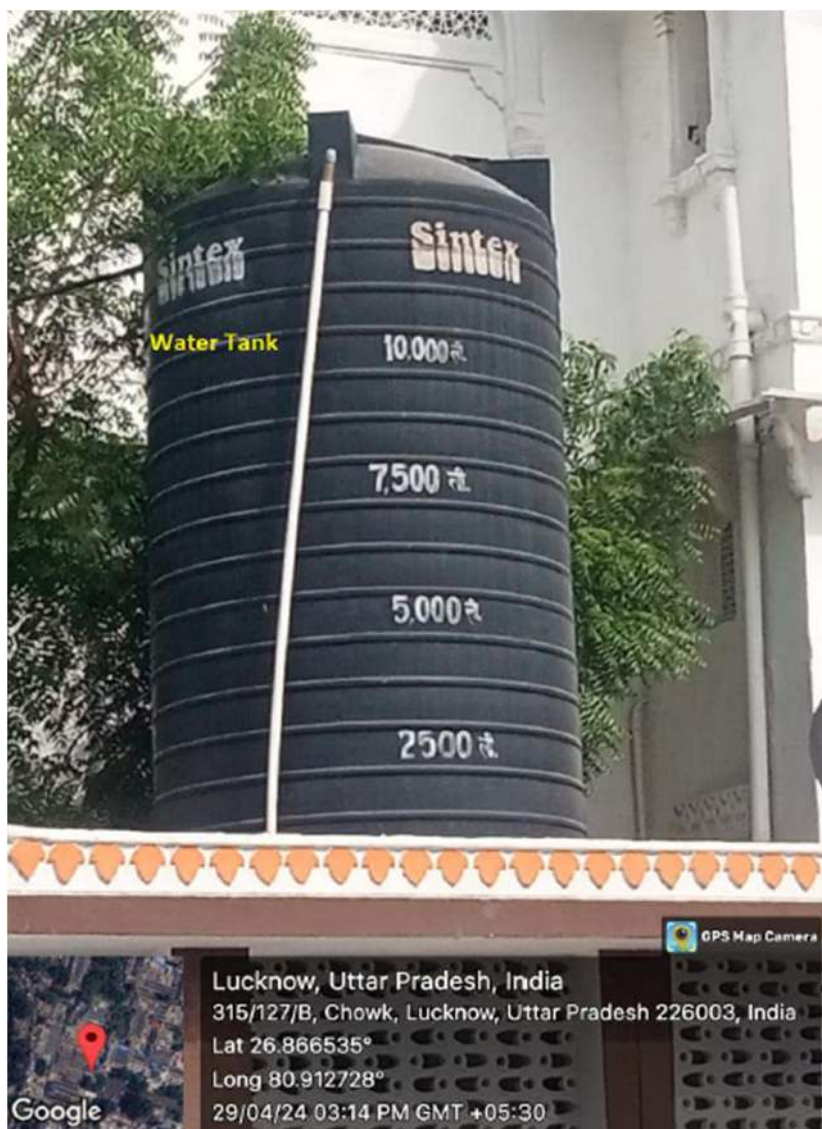
Roof top of water tank use to store water for further distribution
