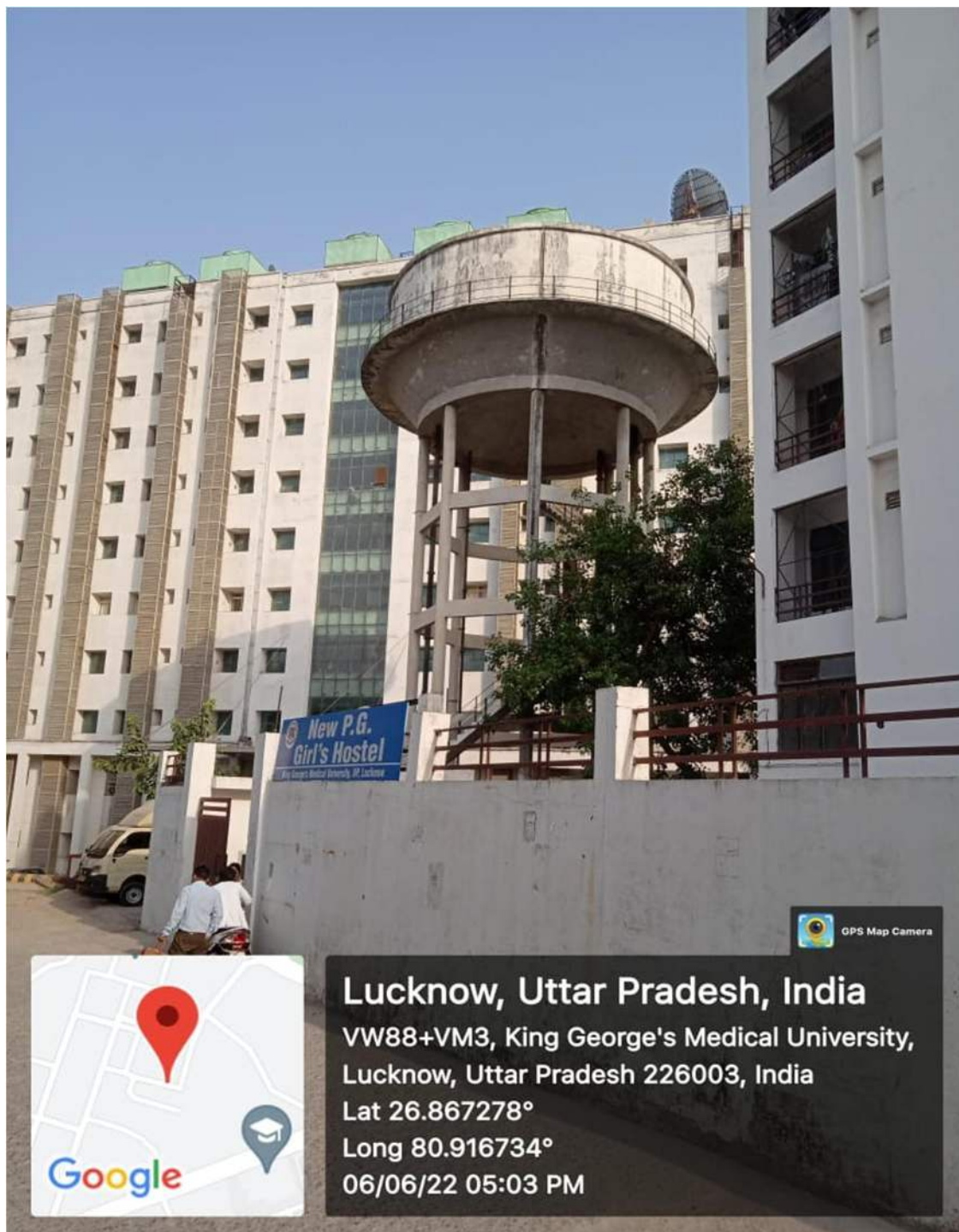
Overhead water tank use to store water for further distribution
