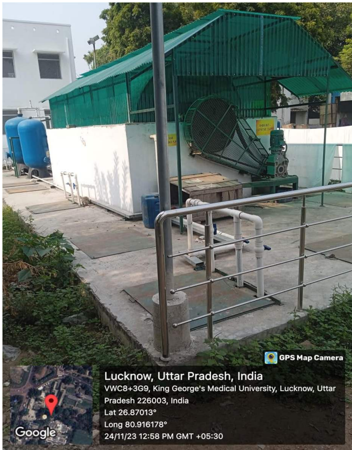
Sewage Treatment Plant behind Mortuary
